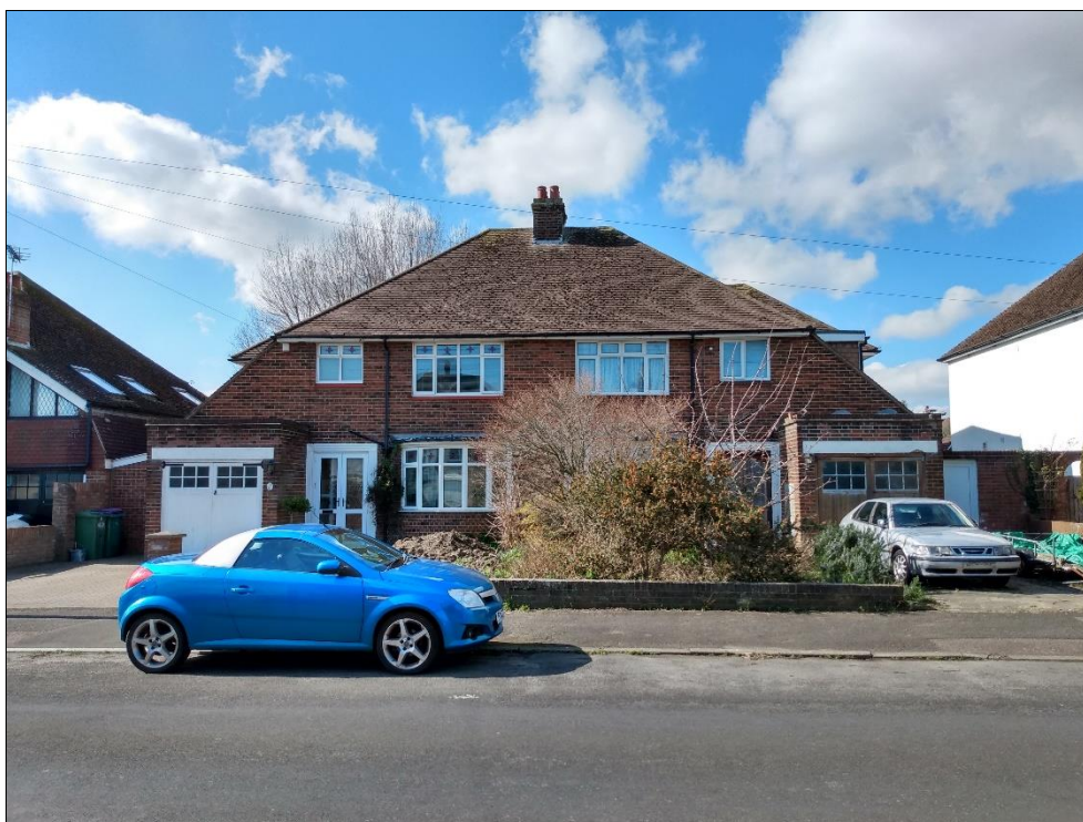
Figure 8: Frontage of nos.32 and 34
